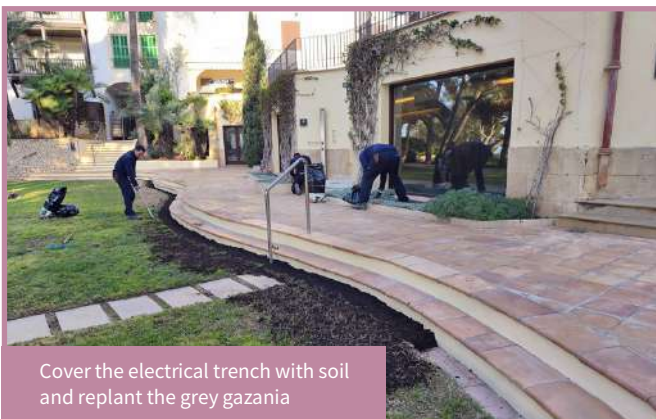
Touch-ups in Restaurant
